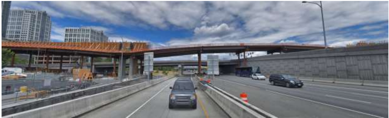
Figure 64: Falsework of Sound Transit's guideway structure on I-405 southbound traffic, looking north (photo credit to Google Map, Oct 2018).
