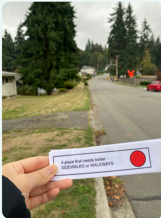
An example of a missing sidewalk
