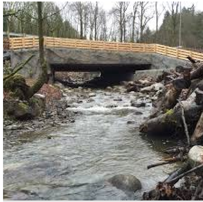
Coal Creek Parkway Culvert
