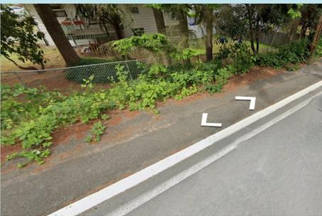
**North Side:** Pre-existing but non-compliant sidewalk. Steep slope into houses and fences on the northern edge, may need wall. Sidewalk curb acts as road line.
