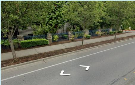
**North Side:** Six-foot sidewalk, with four-foot planter. Shoulder is not currently wide enough for a 5-foot bike lane.
