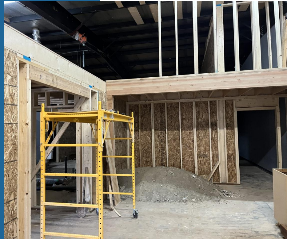
Theatre33 construction in BelRed.
