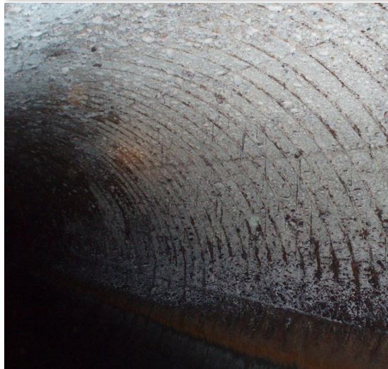
South Interceptor (Renton, located under I-405)
