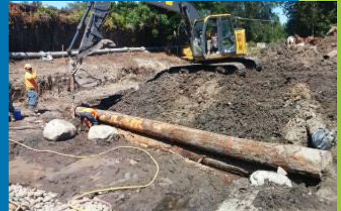
Richards Creek Channel Improvements
