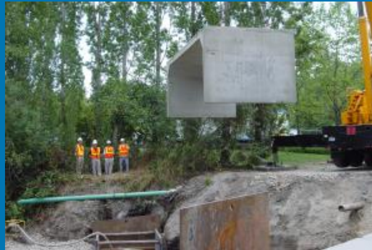
Bannerwood Park culvert
