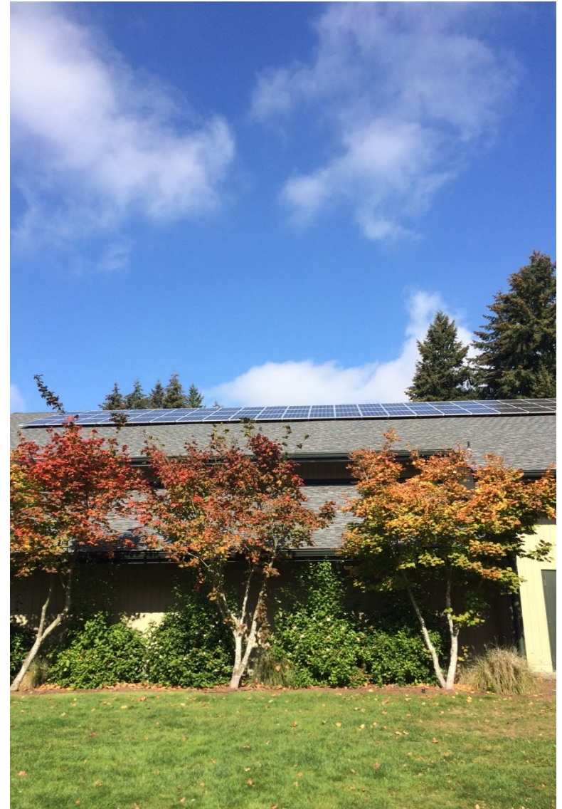
Solar array on Crossroads Community Center.
