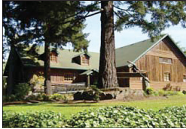
Existing Highland Park and Community Center.
