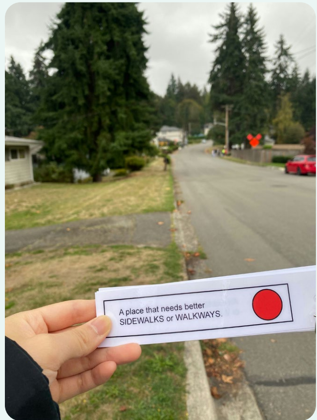
An example of a missing sidewalk
