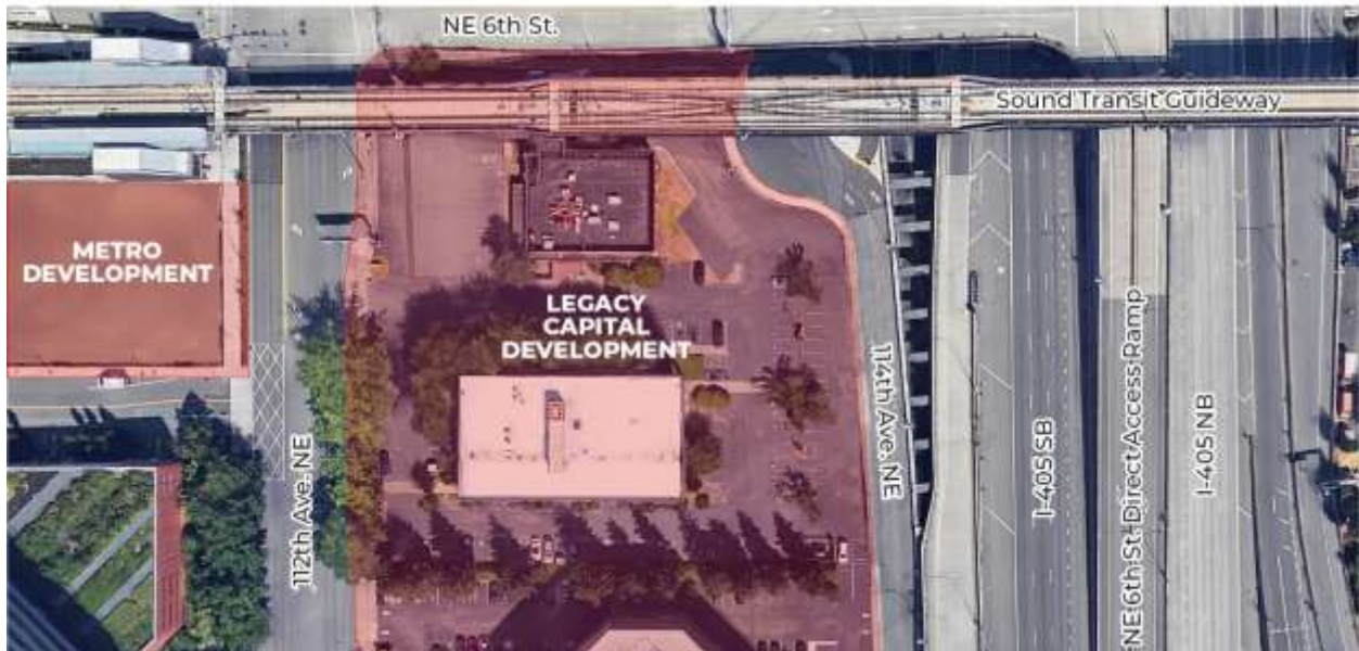
Figure 22: West of I-405, including the east portion of the Metro Legacy sites (background image credit: Google Maps).
