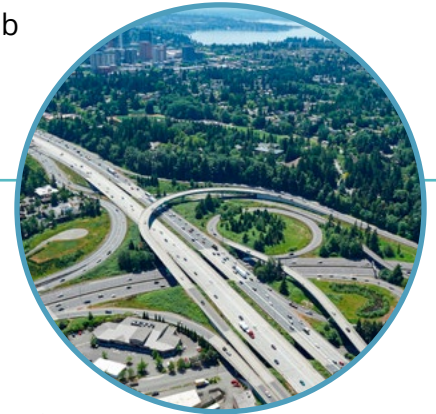
Aerial of I-405 and the SR 520 Interchange
