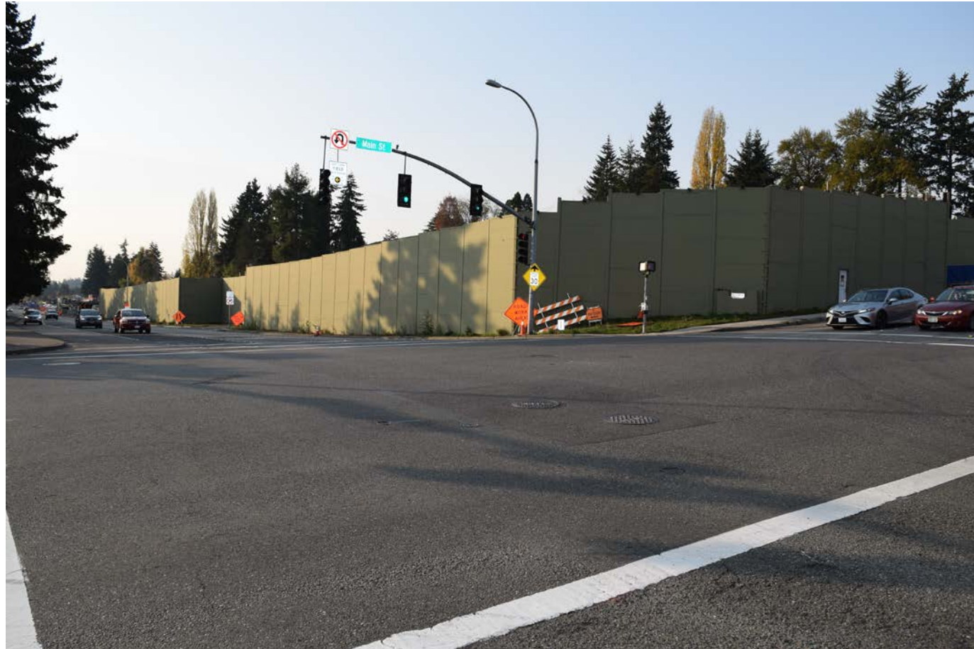
Temporary Sound Wall at South Portal
