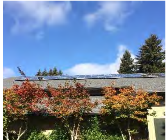
Photo: Crossroads Community Center Solar Array
