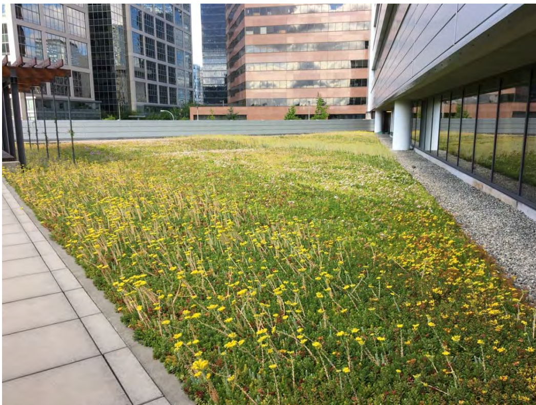
Photo: Bellevue City Hall Green Roof.
