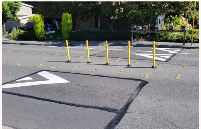
Figure 5: One of the three speed cushions implemented along 119th Avenue Southeast in 2023.
