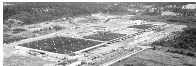
A Safeway distribution facility in BelRed, formerly a Japanese American farm, was torn down to build the Spring District.*
