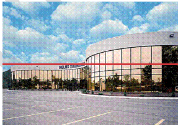
Unarticulated roof lines.
