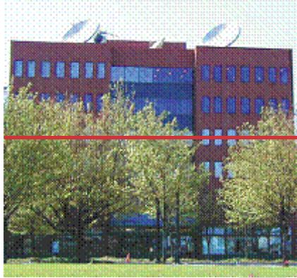
Rooftop telecommunications equipment visible from public spaces.
