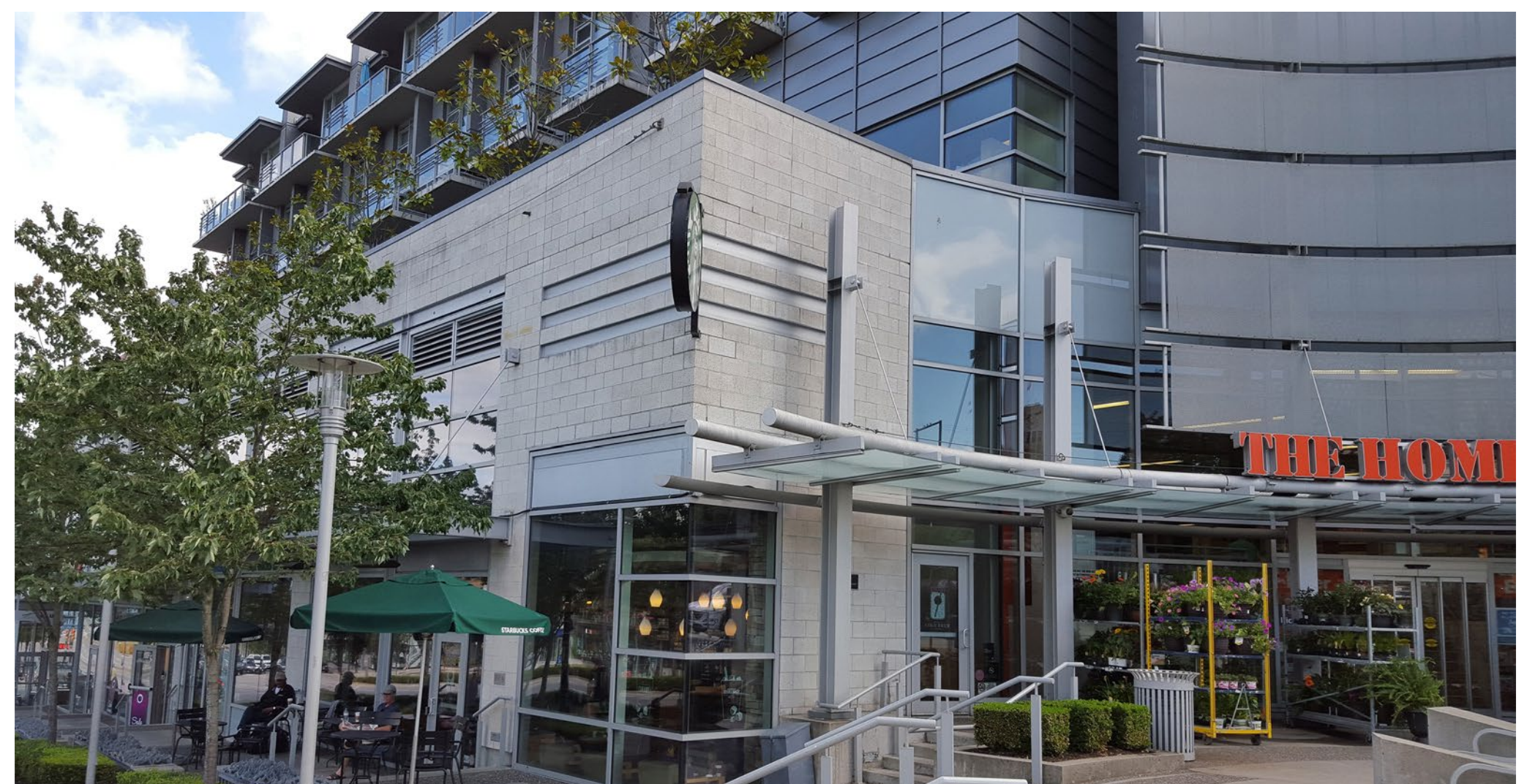
Large-format commercial space can be designed to fit within a mixed-use, urban environment.
