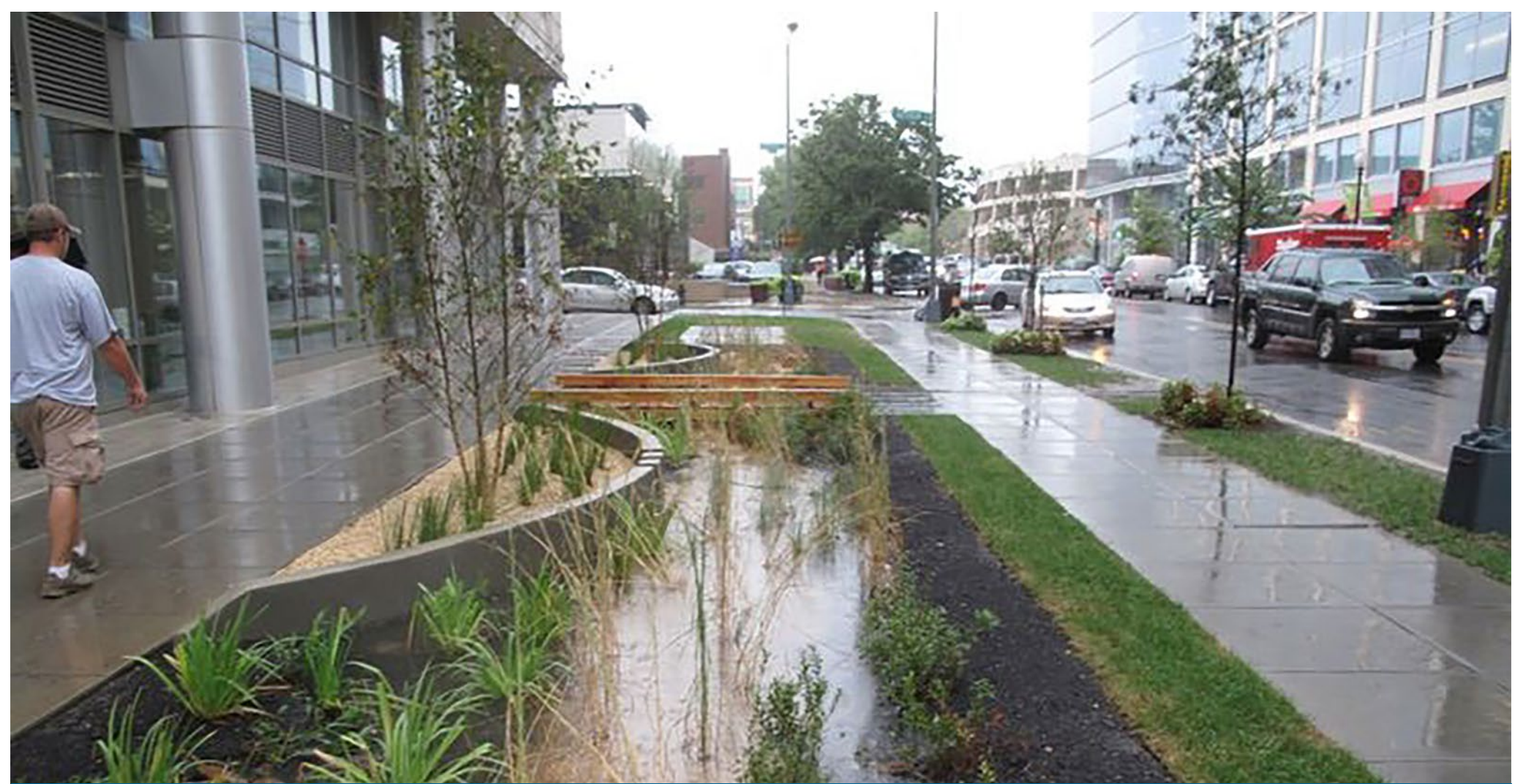
Green street infrastructure adds visual interest, provides a buffer between cars and pedestrians, and helps manage stormwater runoff.
