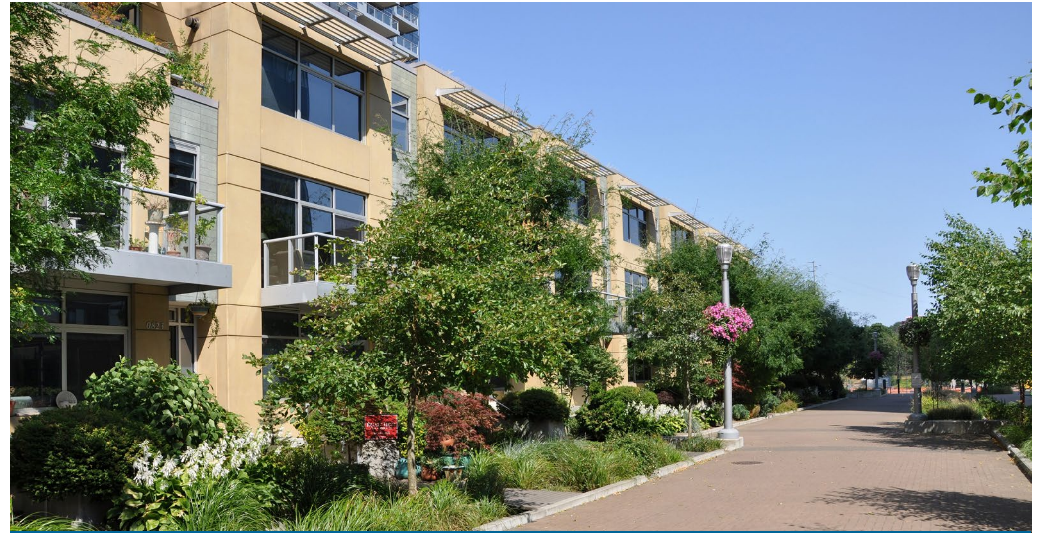
Street-facing units can add to neighborhood character, vibrancy, and sense of safety.
