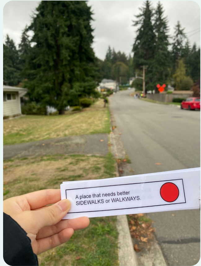
An example of a missing sidewalk
