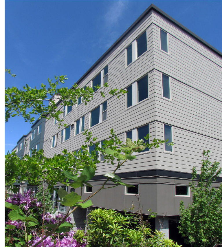
30Belleuve at St. Luke's Church, Imagine Housing – Northwest Bellevue; 62 one, two and three bedroom affordable apartments, average unit size 605 sqft.; 14.3 dwellings per acre; R-20 zone.
