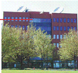
Rooftop telecommunications equipment visible from public spaces.
