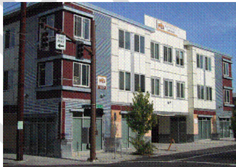
Simple entrance flush to façade without articulation.
