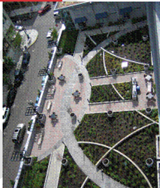
Attractive rooftops well integrated into overall building design.
