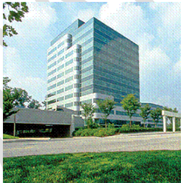
Unbroken volume of building that does not enhance the street environment and lacks human scale.
