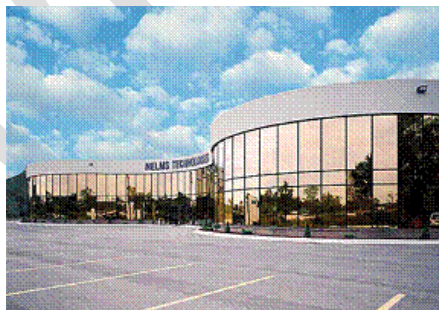
Unarticulated roof lines.
