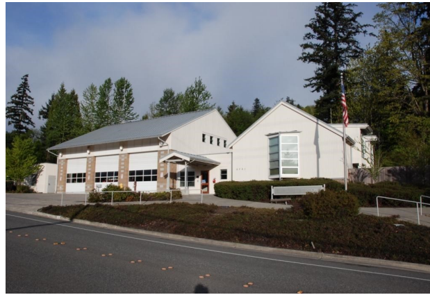
Bellevue Fire Station Eight
