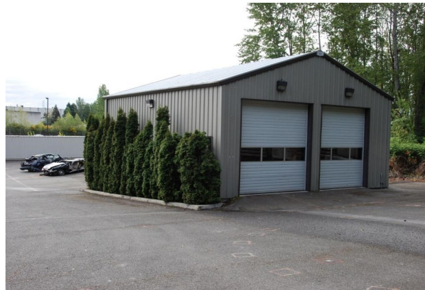
Bellevue Fire Training Center—Garage
