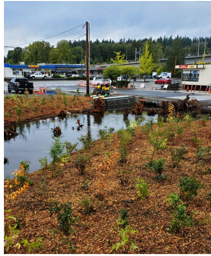
Culvert replaced at Valley Creek across NE 21 st Street
