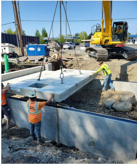
Culvert replaced at Valley Creek across NE 21 st Street
