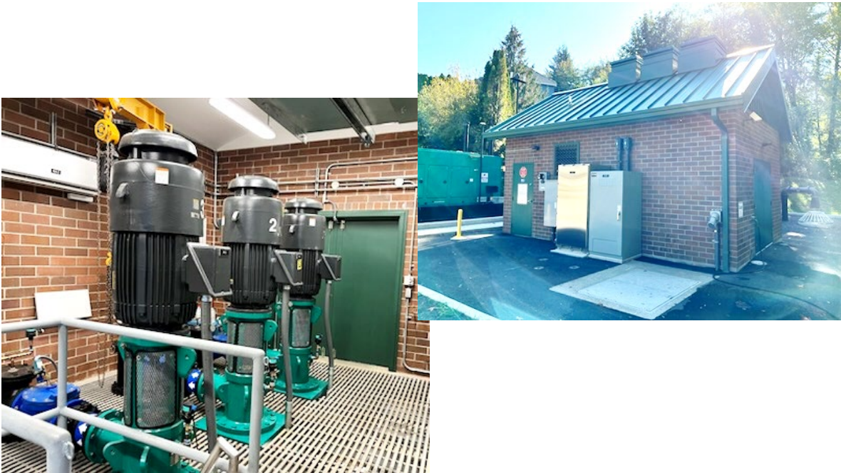
(Cougar Mountain 1 Pump Station, constructed in 2025)
