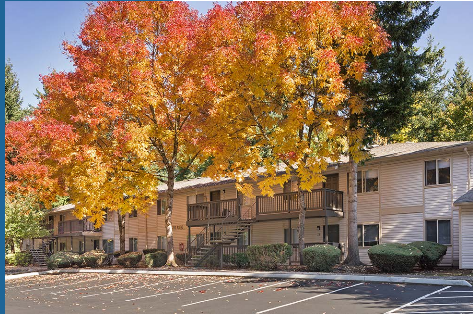
KCHA Kendall Ridge. 240 units Preservation
