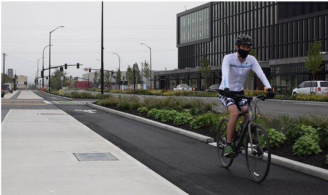
Protected bike lane along NE Spring Blvd provides safe and reliable route for cyclists
