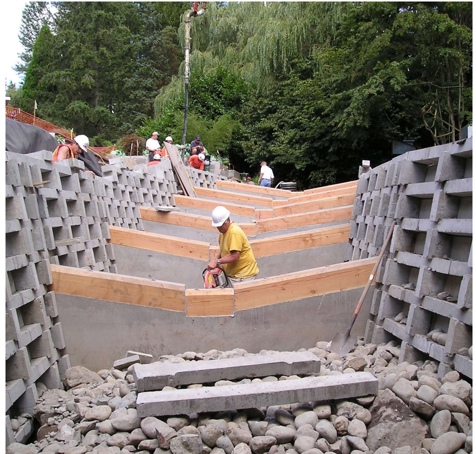
Mercer Slough fish ladder
