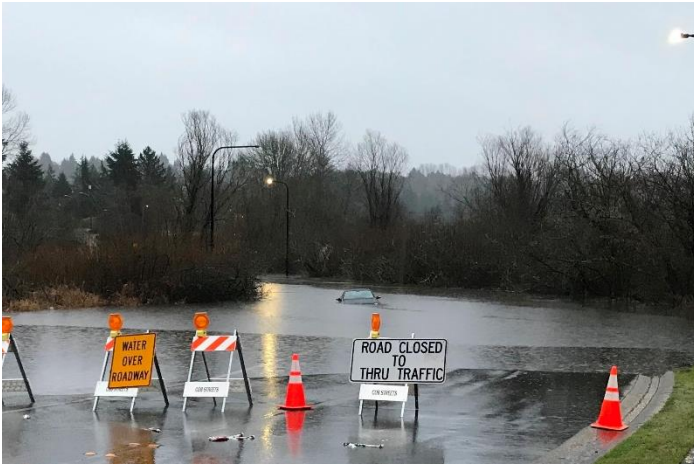
Flooding Event (SE 7 th Pl in Wilburton)
