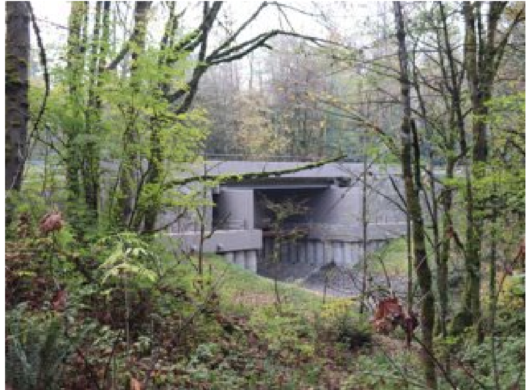
Lakemont Blvd. Emergency Bridge Project
