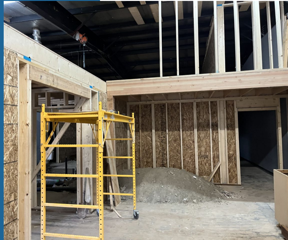
Theatre33 construction in BelRed.
