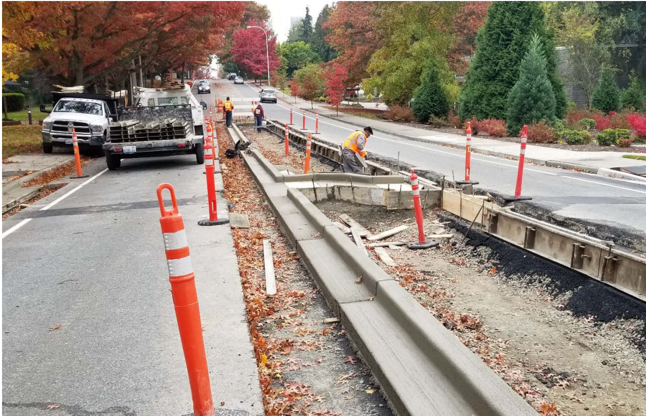
112 th Ave NE crosswalks, medians, bike lanes and maintenance
