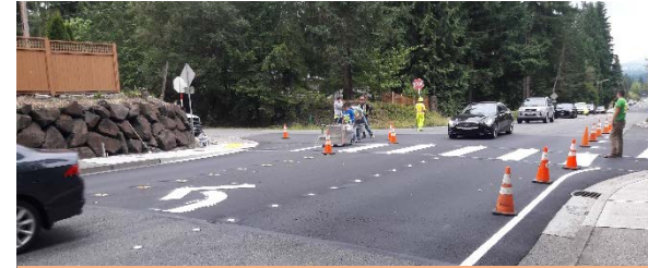
156 th Ave SE crosswalks
