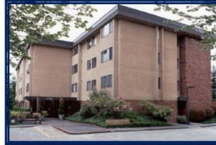
59 units (1 bedrooms) Mercer Island
