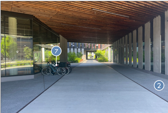
Between NE 14th Terrace and NE Spring Blvd (Spring District, Bellevue)
