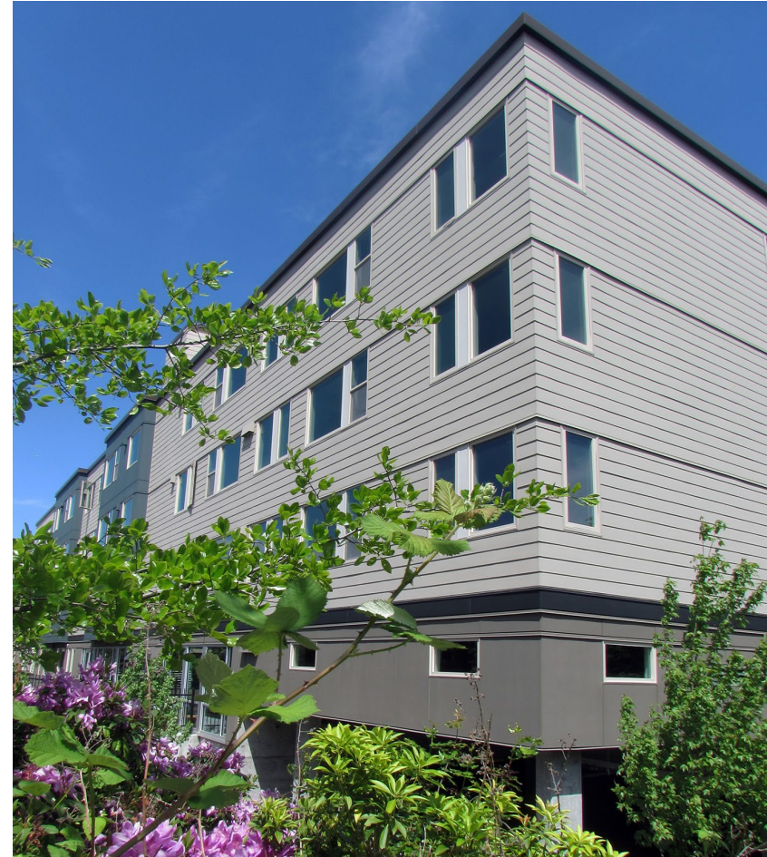
30Bellevue at St. Luke's Church, Imagine Housing – Northwest Bellevue; 62 one, two and three bedroom affordable apartments, average unit size 605 sqft.; 14.3 dwellings per acre; R-20 zone.
