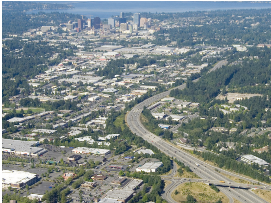
View of Bel-Red Subarea looking west.
