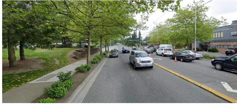
Type M curb (Mv subtype) Bellevue, WA 116 th Avenue NE
