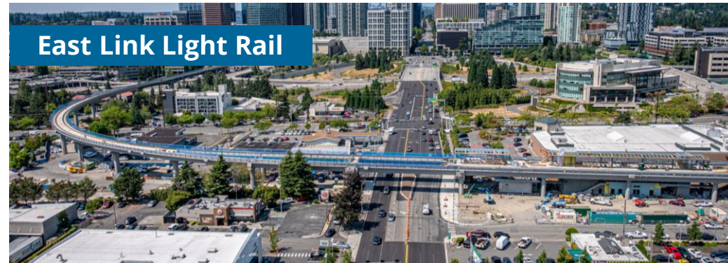
East Link Light Rail
