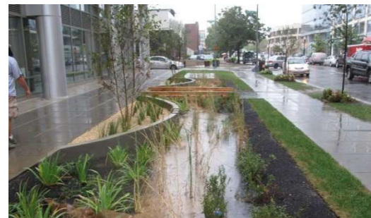
Example image used during engagement to highlight policy moves around green stormwater infrastructure and vegetation in the TOD area.
