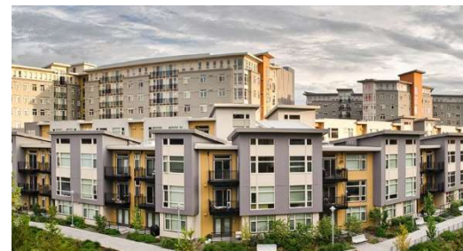
Example image used during engagement to highlight policy moves around building densities that include a range of high-rise and mid-rise development that transitions to residential areas to the east.
