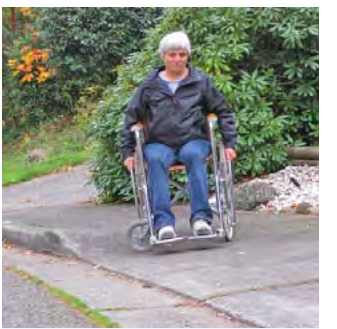
Steep driveway cross slope.
