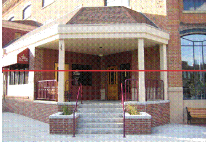
Visual and physical obstructions such as recessed entryway and grade separation.
