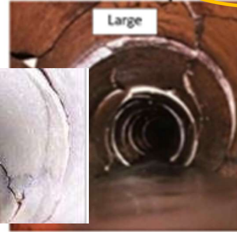
Fracture - Multiple (FM)
