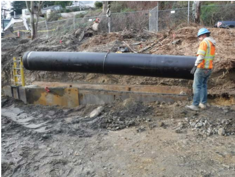
Gravity Sewer Line via Open Cut Construction
