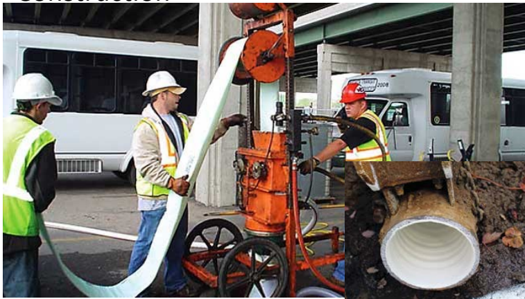
Cured-in-Place Pipe (CIPP)
