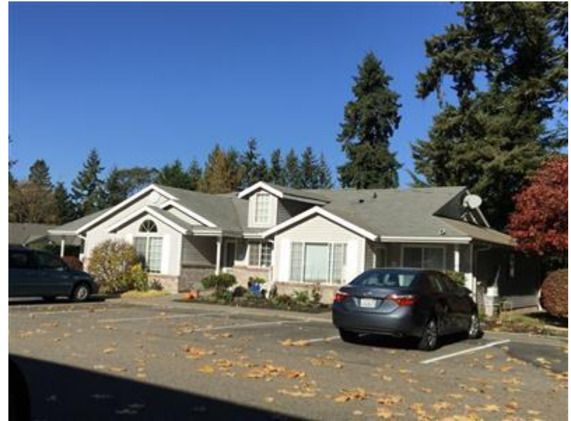
Cambridge Court – Senior Housing – Church of the Resurrection – Lake Hills 12 affordable units in 6 duplexes
