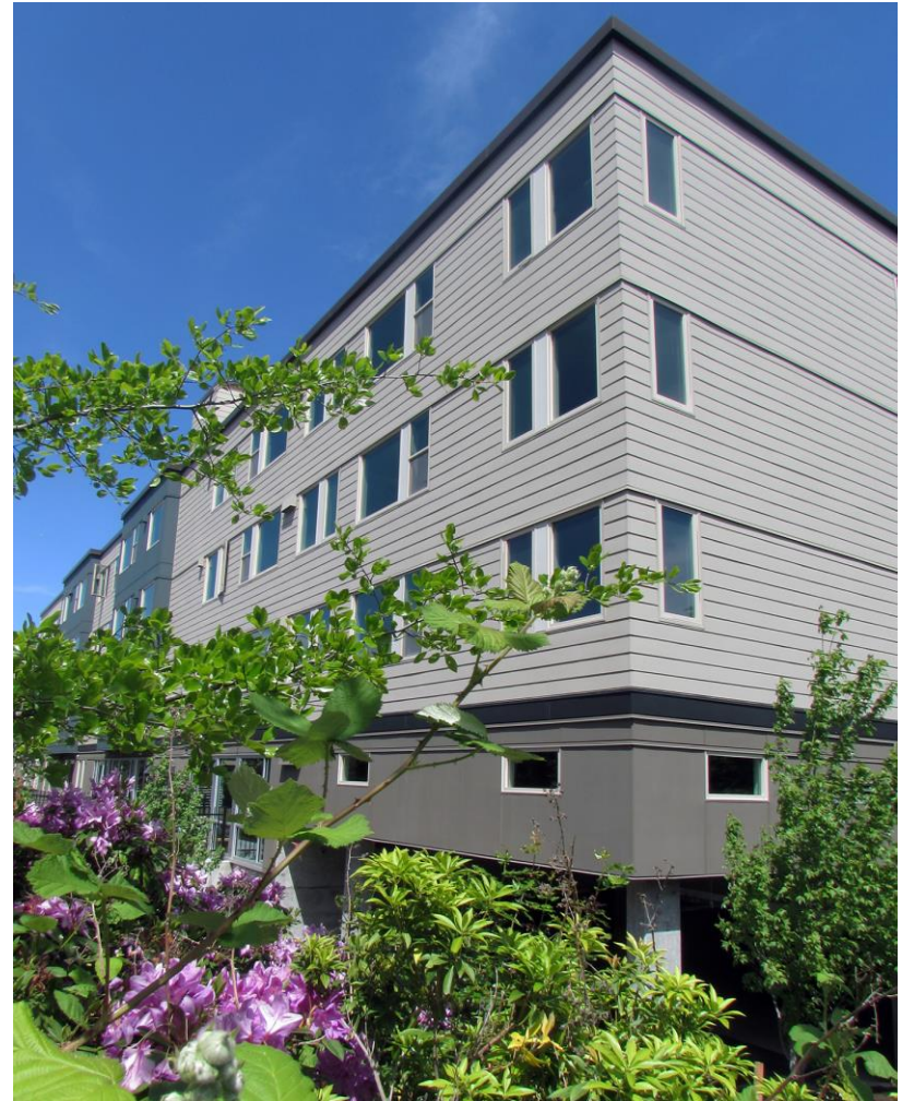
30Bellevue at St. Luke’s Church, Imagine Housing – Northwest Bellevue; 62 one, two and three bedroom affordable apartments
