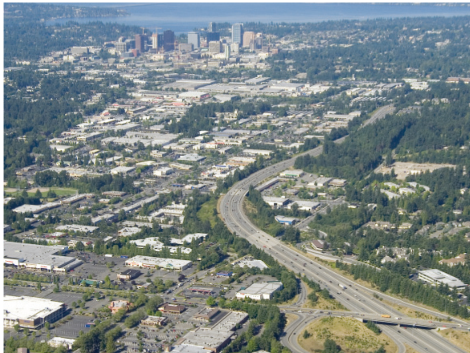
View of Bel-Red Subarea looking west.
