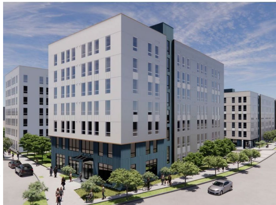
Bridge Housing project at OMFE
