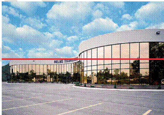
Unarticulated roof lines.
