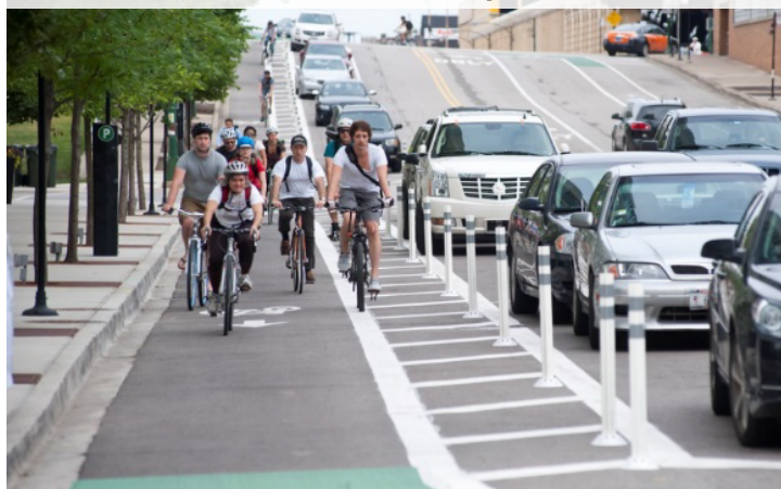
Parking, Painted Buffer, and Post Separation
