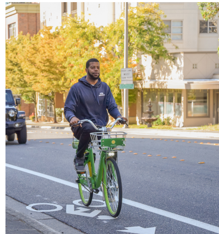
Figure 9. A person riding northbound in the striped bike lane south of NE 2nd St, where the street is only wide enough to provide a painted buffer in the southbound direction.
