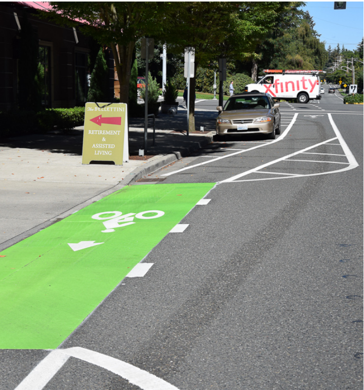
Figure 6. Green markings installed where the bike lanes pass by high-traffic driveways call the attention of people driving and bicycling to be alert through areas where their paths cross.
