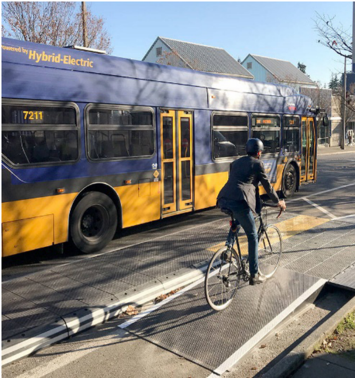
Figure 3. The new bus platform is installed on 108th Ave NE south of NE 2nd St. It is made of 300 interlocking plastic panels that snap together, allowing for its rapid installation.
