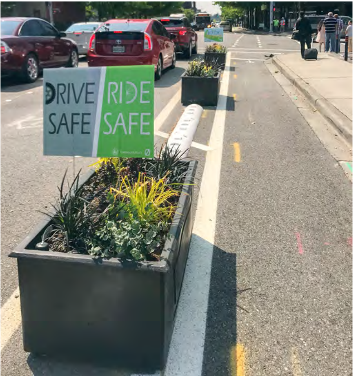
Figure 5. Planter boxes were installed in the painted buffer area along several segments of the demonstration bikeway, providing a decorative form of enhanced physical separation.
