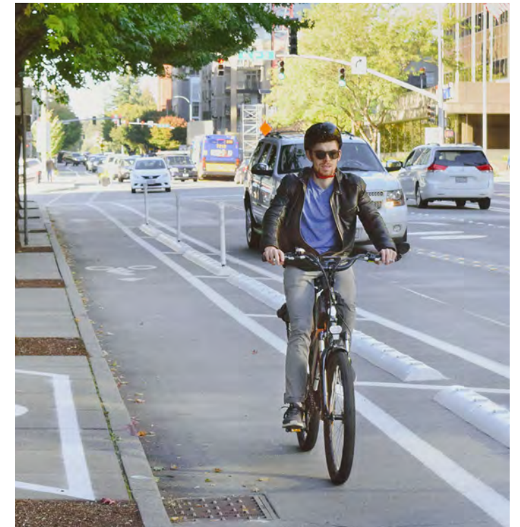
Figure 8. A person riding southbound in the bike lane south of NE 8th St, where Tuff Curb—a durable traffic safety product—provides physical separation for people on bikes.
