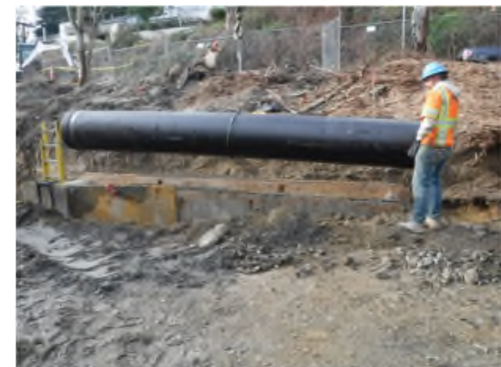
Gravity Sewer Line via Open Cut Construction
